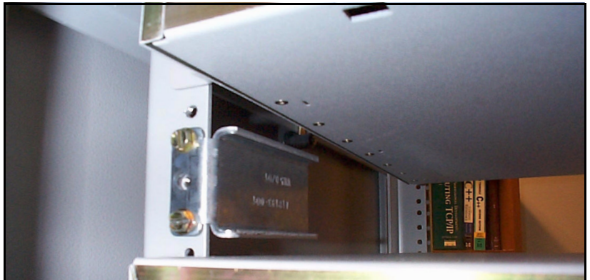
Installed rack-mount bracket
