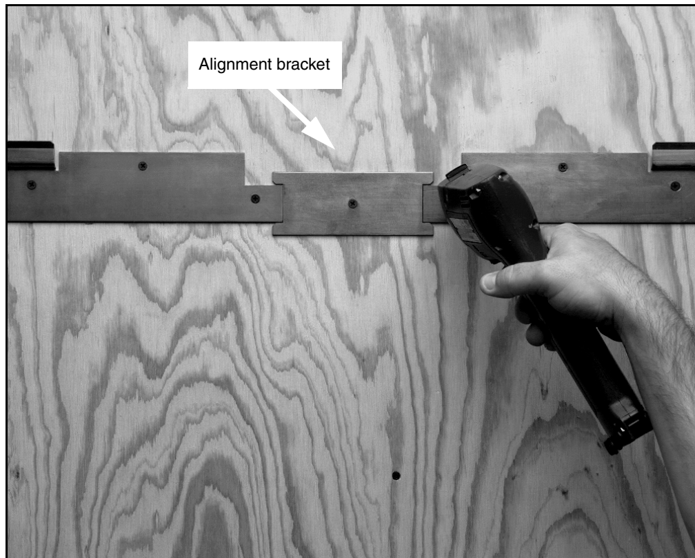
Figure 35 Brackets for horizontal expansion
